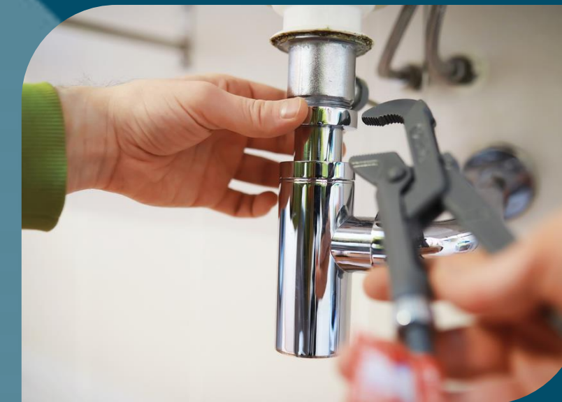
MINOR PLUMBING REPAIRS
